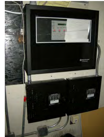
The development's central fire alarm control panel
