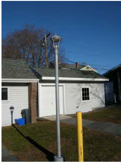
Example of new fluorescent site lighting fixture
