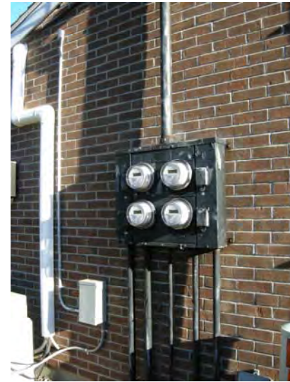
Typical original meter box station
