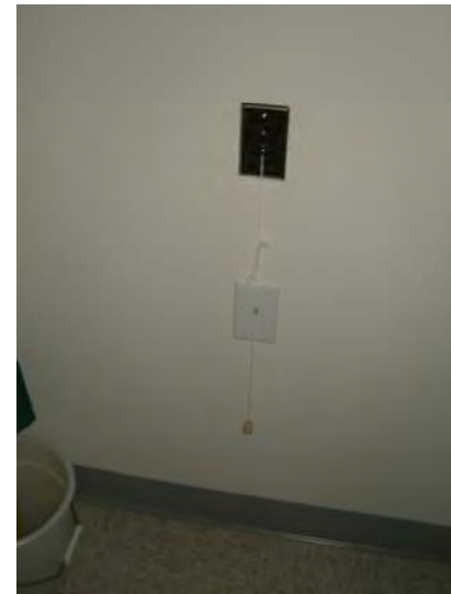
Typical in-unit emergency-call pull station. Connected to central system
