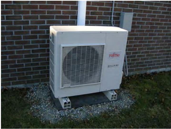
The exterior condenser section of the community building's ductless heat pump
