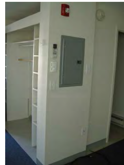
Typical one-bedroom unit recently replaced circuit breaker panel, horn/strobe, and smoke detector
