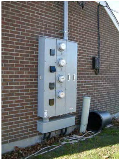
Typical upgraded meter box station
